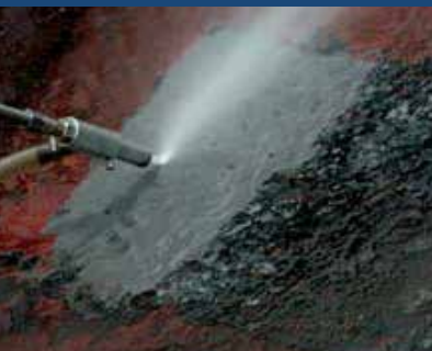
Surface - Sand Blasting
