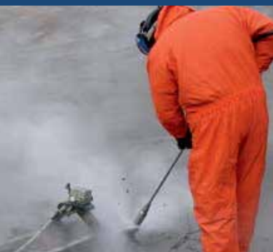
Removing concrete
